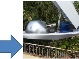
Magnetic Ballast, Igniter, Capacitor
